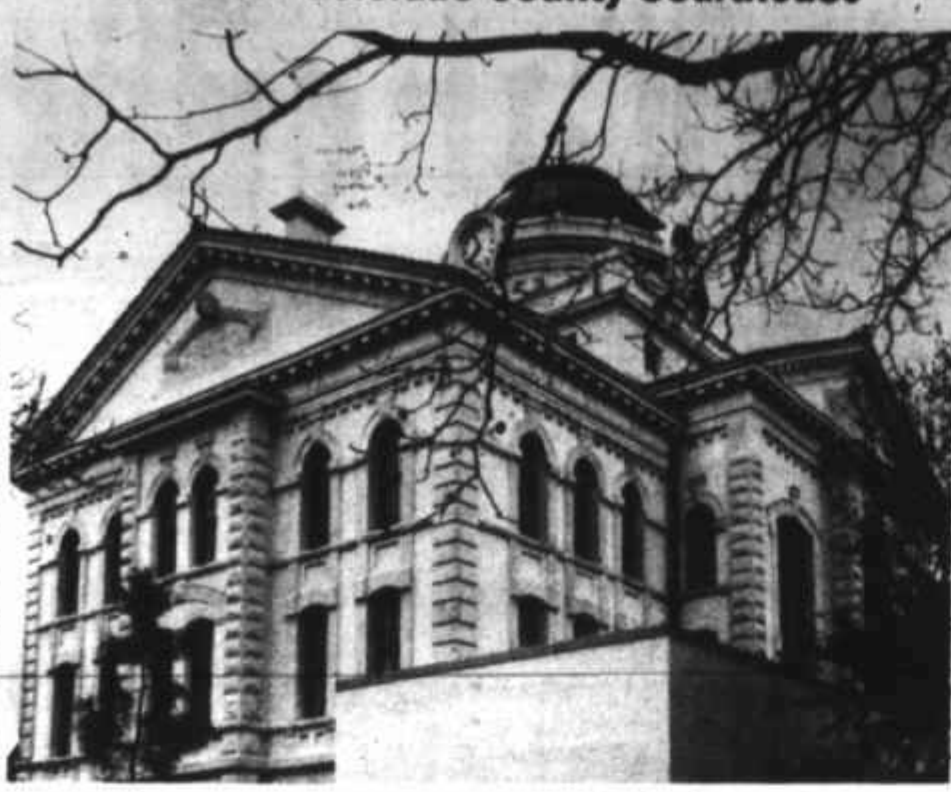
Colorado County Courthouse, built in 1890 will be open to the public during the 21st Annual Magnolia Homes Tour in Columbus, Saturday and Sunday, May 15 and 16. An extensive restoration program, completed early this year, will provide visitors with a view of the beauty and elegance of late 19th century architecture. Homes Tour Photo.
